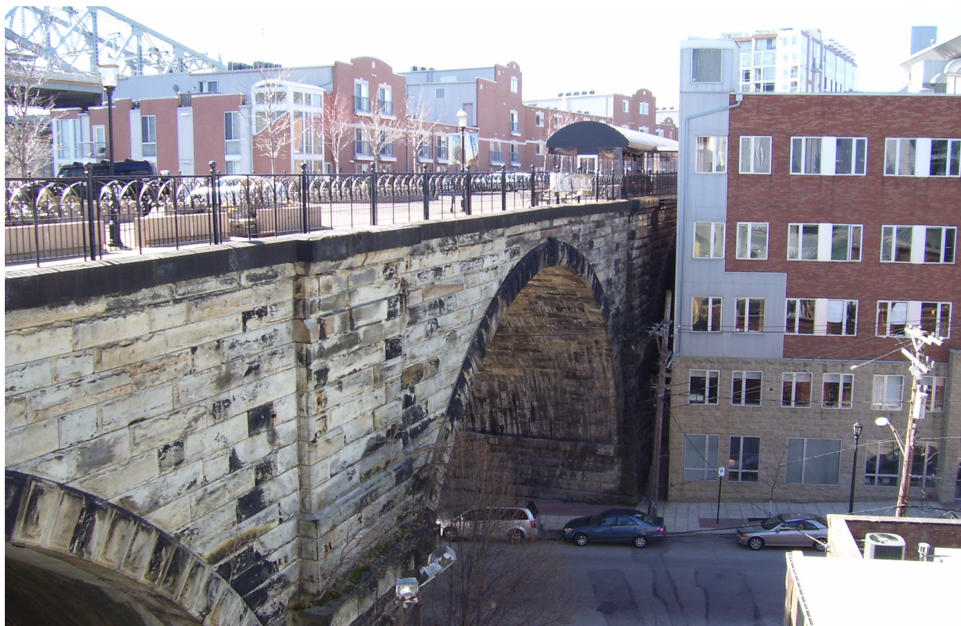
Superior Viaduct in April, 2008 picture by Cindy Spikowski
